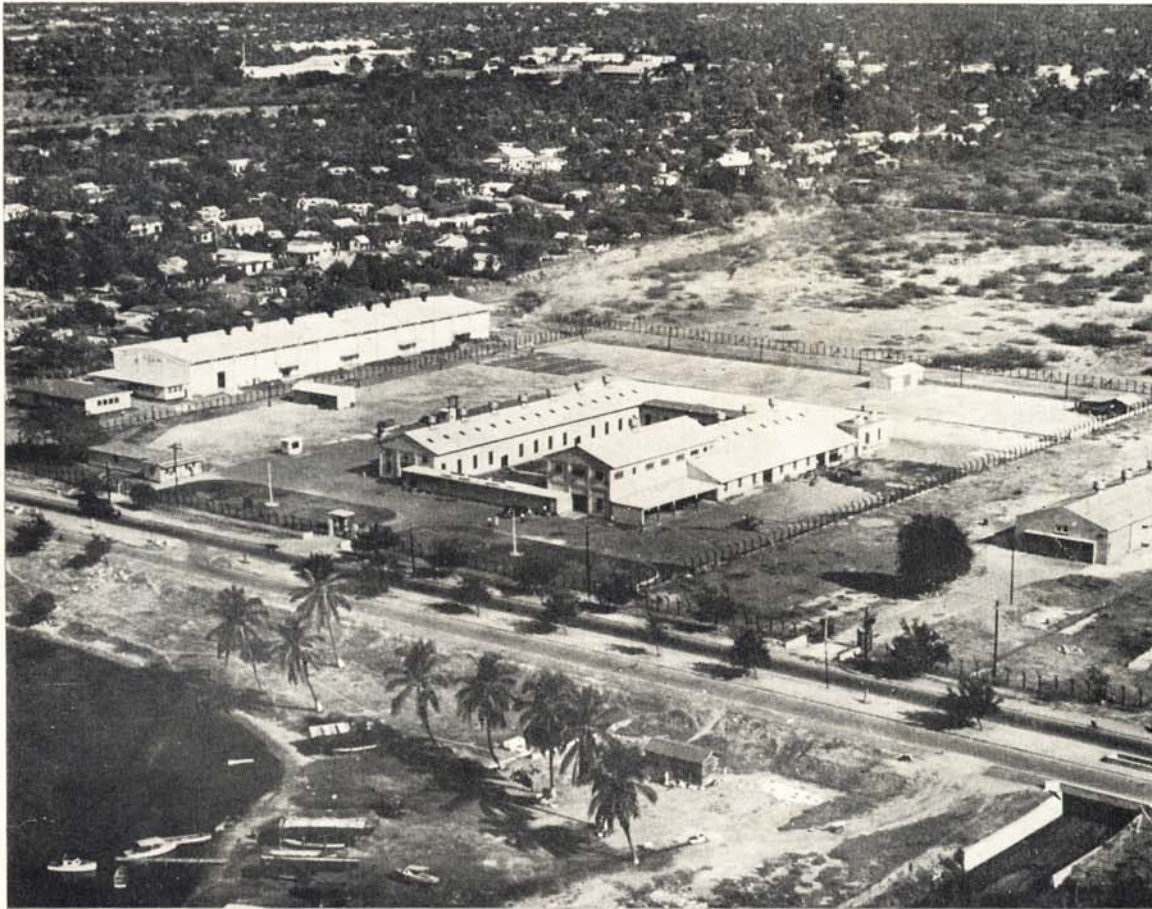
AERIAL VIEW OF THE CENTRAL GRADING AND FINISHING WORKS.
